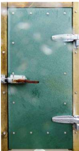
Figure 117 - The galley door
