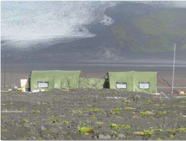
Figure 71 – The completed shelters (operations, dorm)
