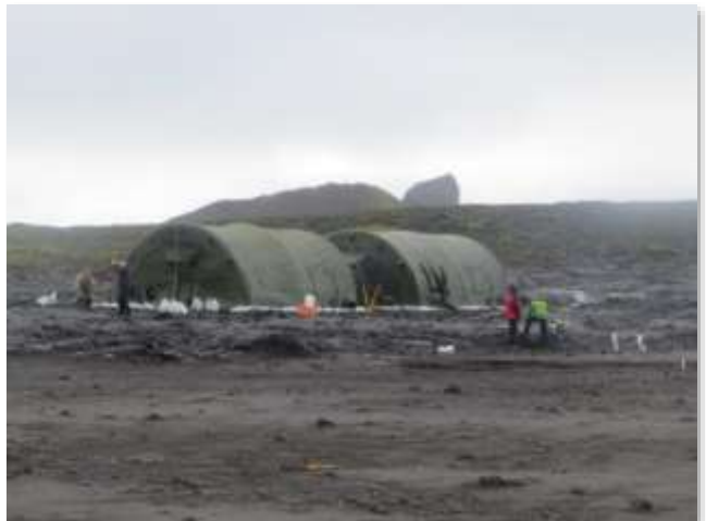
Figure 70 –The shelters are complete.
