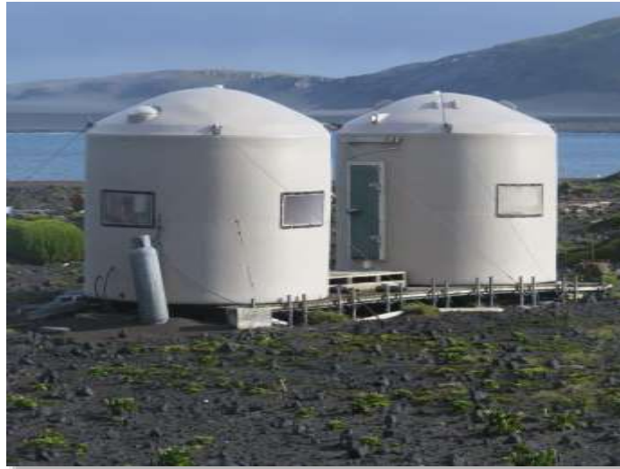
Figure 113 – The AAD refuge shelters, just east of the ANARE ruins
