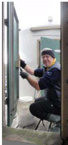
Figure 116 - Repairing the door
