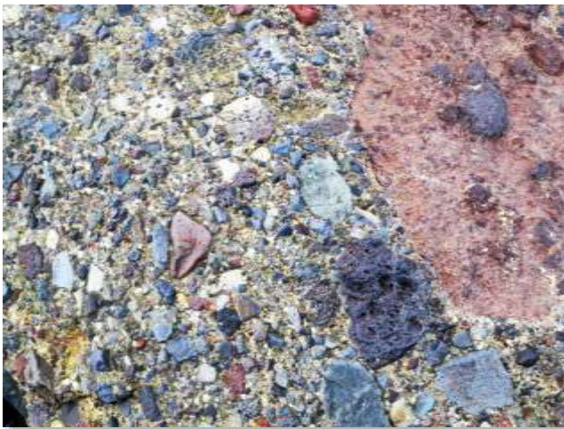
Figure 504 – Detail from previous photo.
