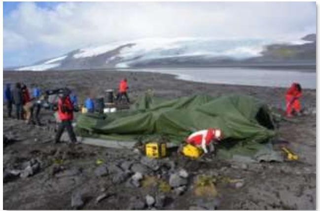
Figure 68 – Inflating the first of two AirBeam shelters
