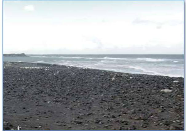
Figure 672 - South breakwater 5 April 2016
