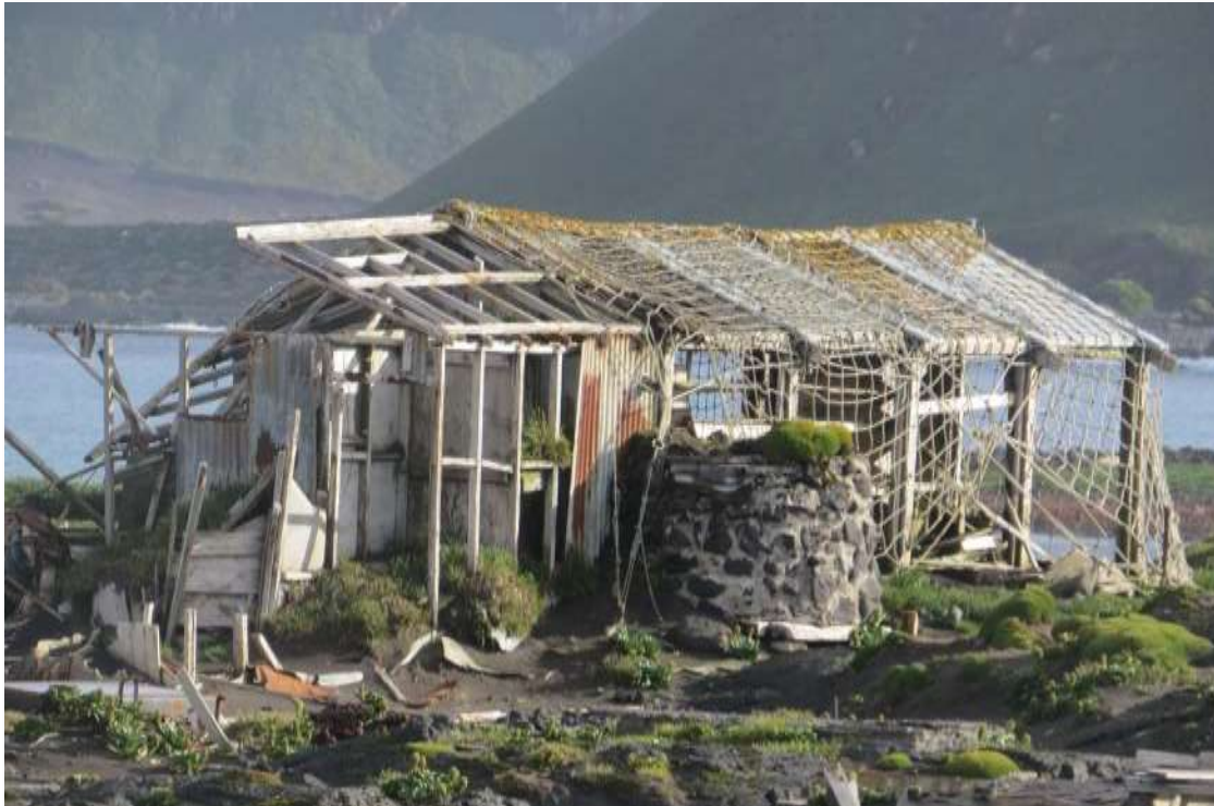
Figure 258 – Ruins of the ANARE station. All pictures on this page were taken from outside the Heritage Zone. ●
