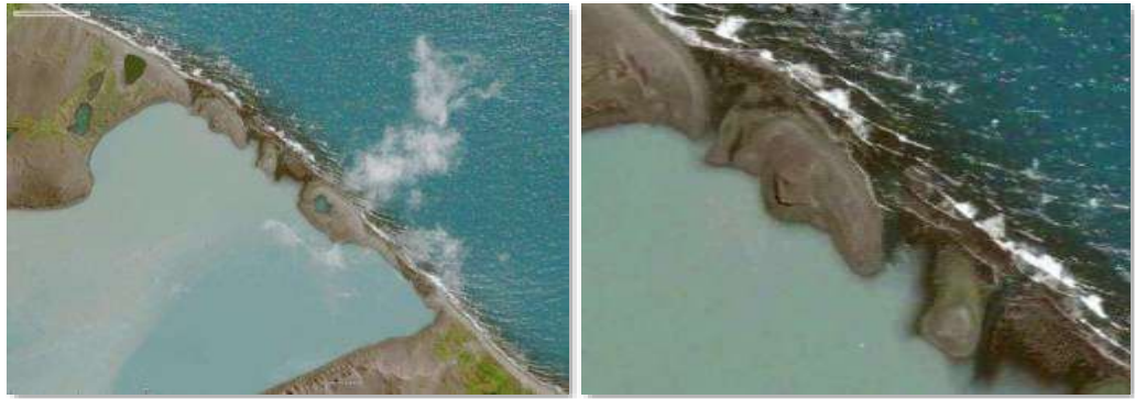
Figure 512 – The north breakwater (satellite 2014) Figure 511 – Detail of the image to left
