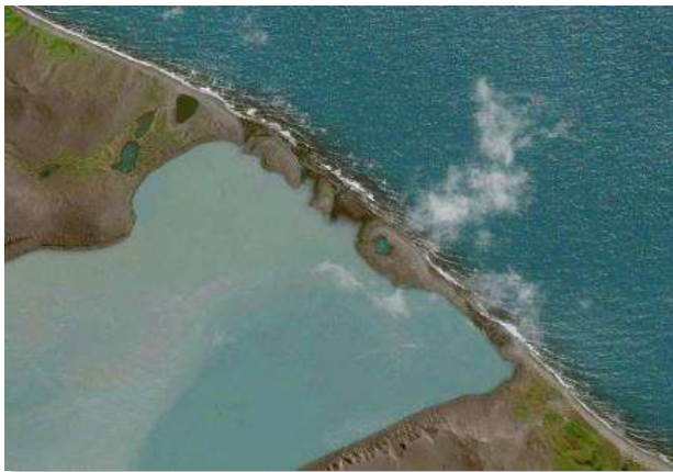
Figure 669 – North breakwater 2007 Satellite image
