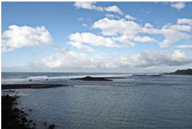
Figure 671 - North breakwater 5 April 2016
