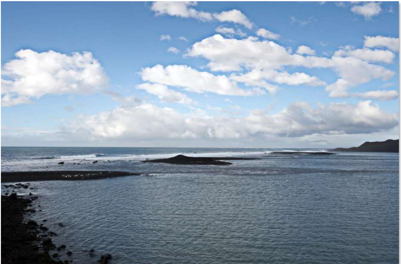
Figure 513 – The north breakwater. Comparing this with the satellite images shows that it is undergoing rapid
